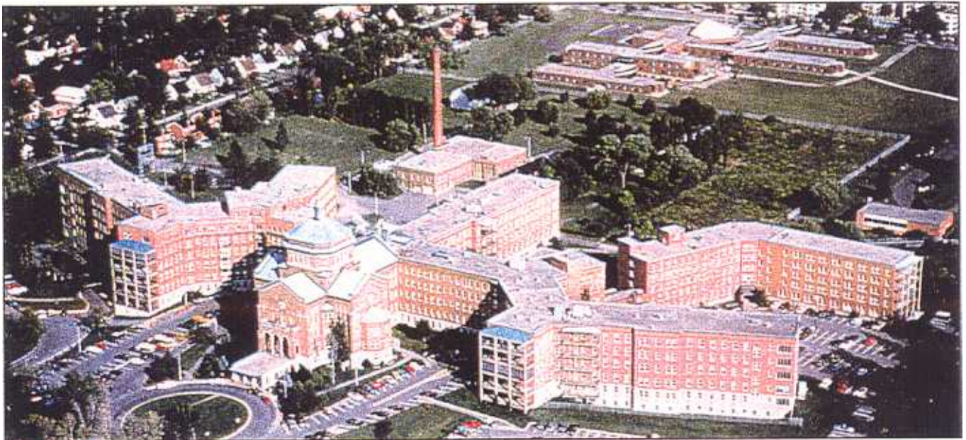
Sacré-Cœur Hospital, Montreal, with the boiler house located at the rear of the building.
